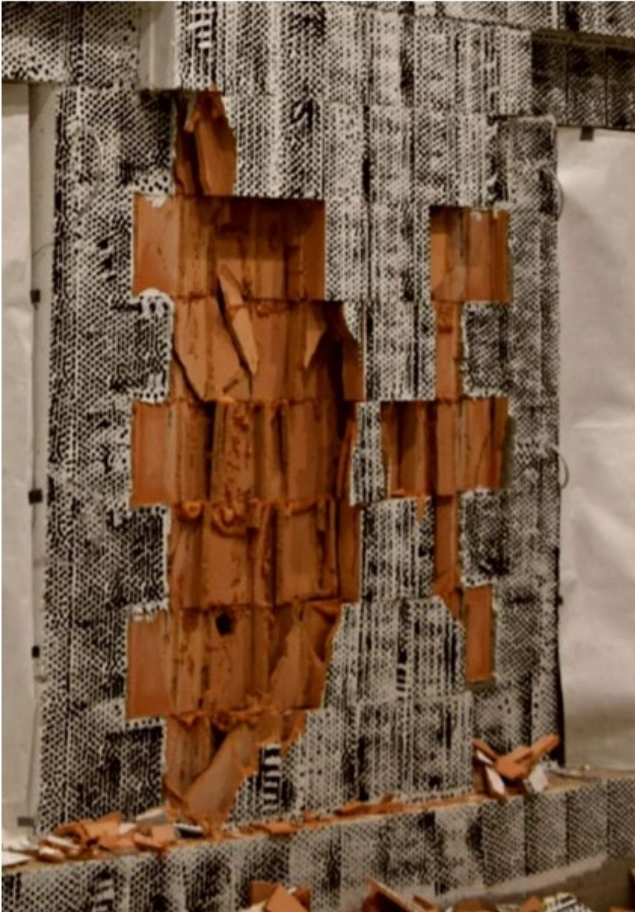
Failure of the pier in the building model
